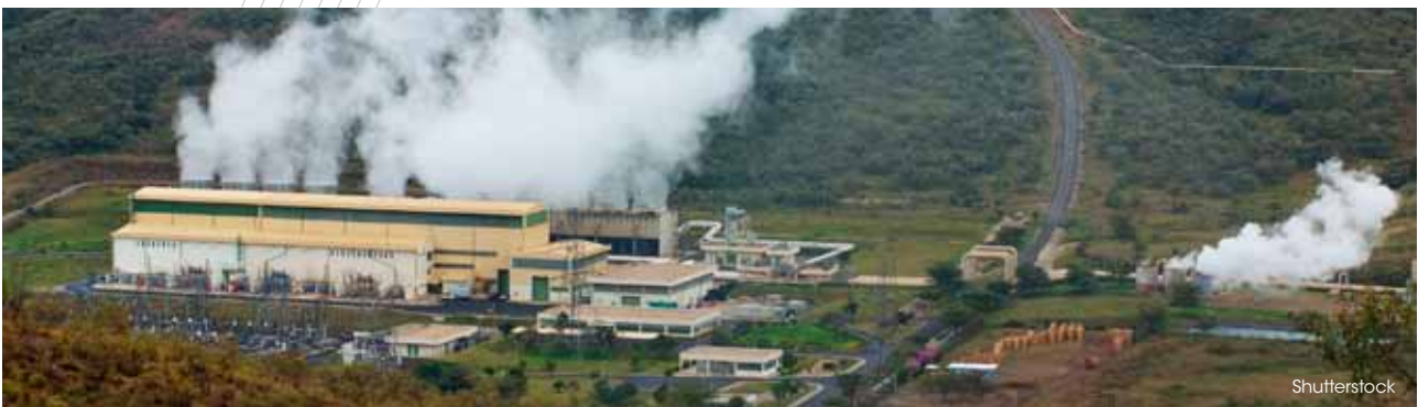
Olkaria Geothermal Plant, Kenya
